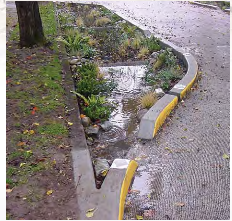
A landscaped curb extension calms traffic and captures and infiltrates street runoff in Portland, Oregon.
